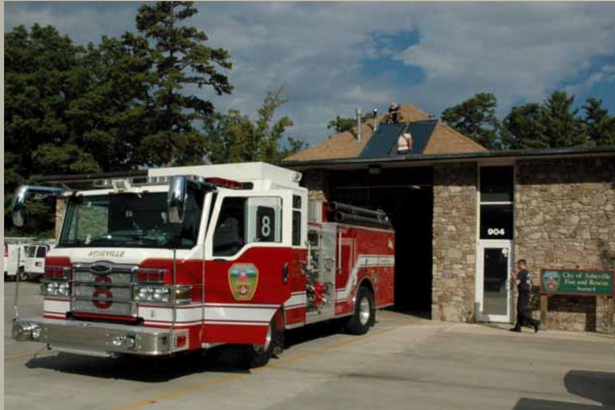
Installation of solar panels on Fire Station 8 in Asheville
